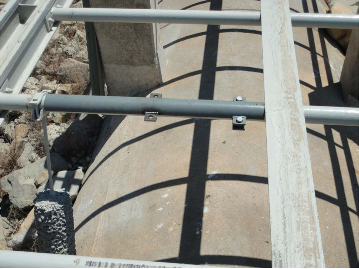
Prototype of cross member adaptor
