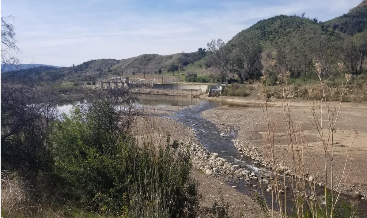
Photograph 1. View of the forebay (facing southwest) following the 2019 sediment removal project (February 4, 2020).
