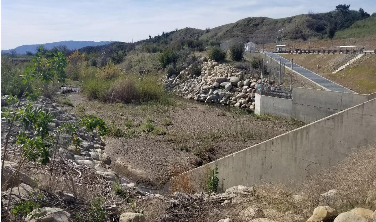
Photograph 11. View of the entrance pool area surrounded by grouted riprap (February 4, 2020).
