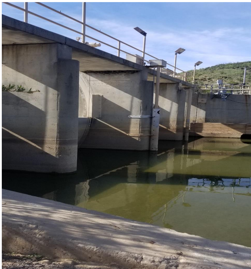
Photograph 6. View of the upstream side of the spillway (February 4, 2020).
