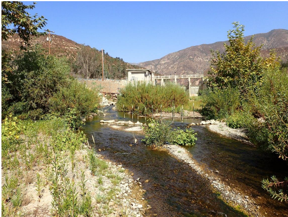
Photograph 6. Sediment deposition downstream of Robles Diversion
