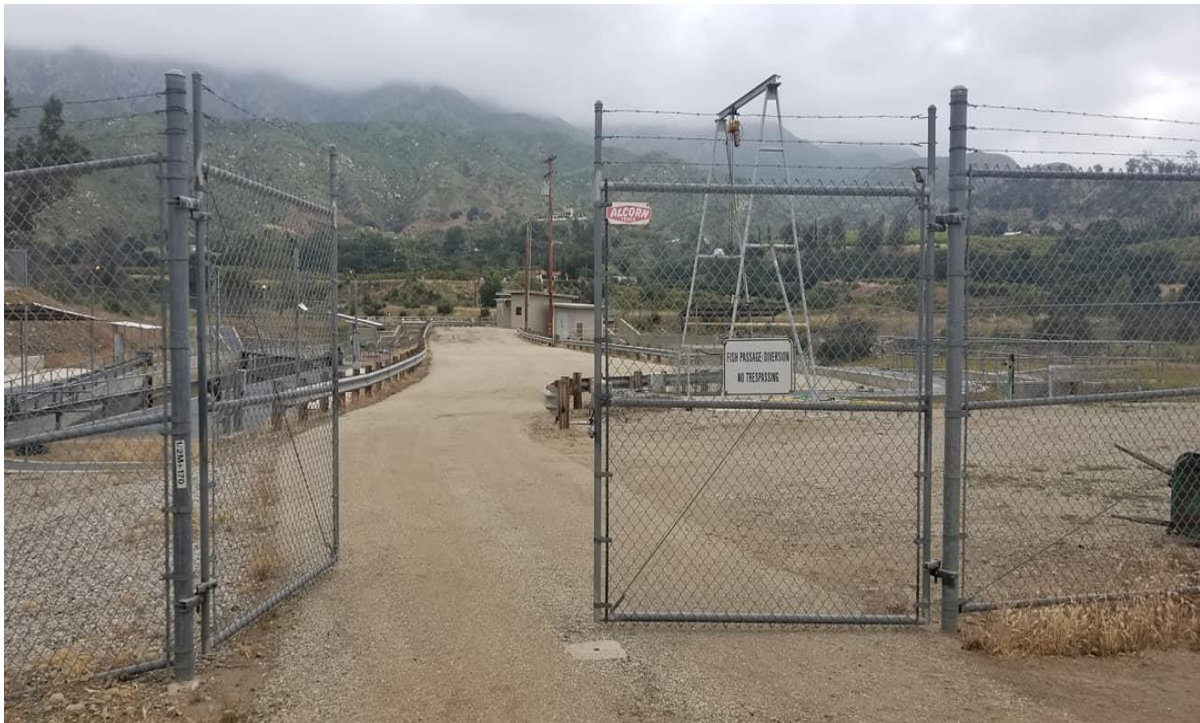
Photograph 14. View of the entrance to the fish passage facility (April 16, 2019).
