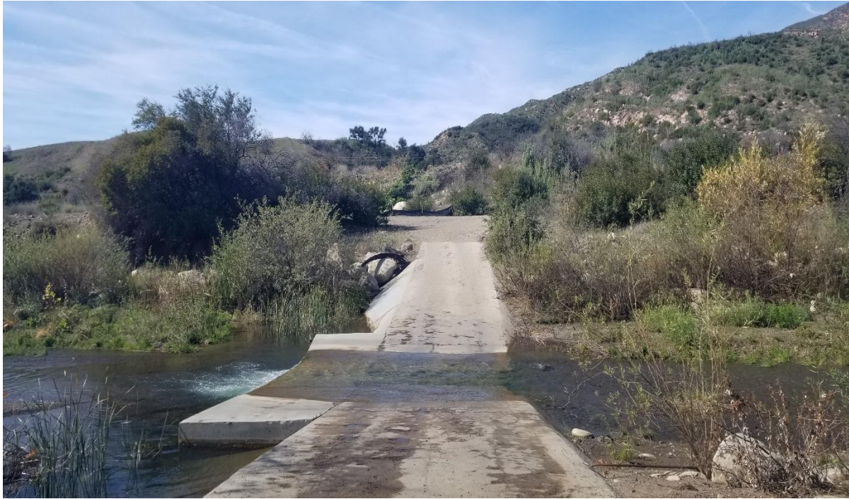
Photograph 13. View of the measurement weir and road crossing (February 4, 2020).
