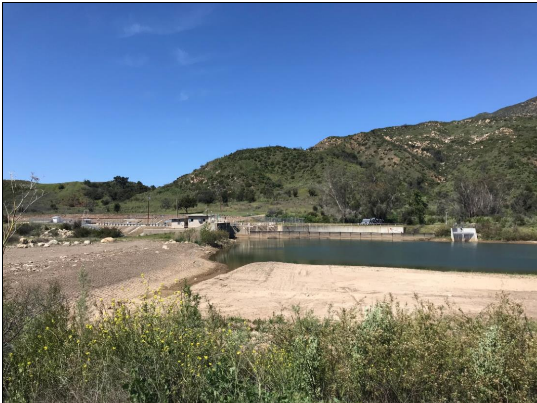
Photograph 1. Overview of Robles Diversion Dam Complex, view northwest. Photo taken April 3, 2020.
