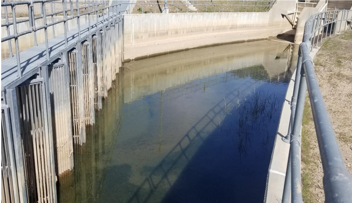
Photograph 5. View of the screenbay looking toward the headworks (February 4, 2020).
