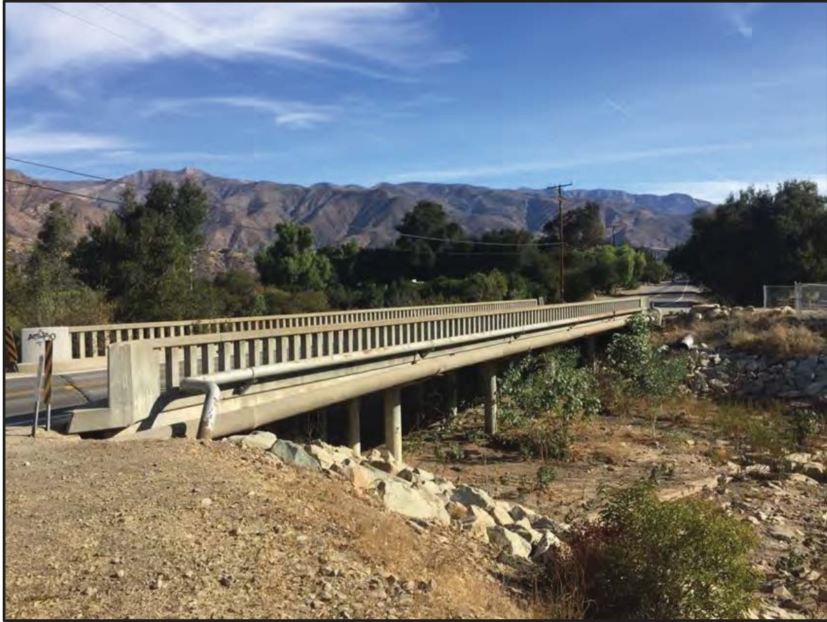
Photograph 1 Pipeline Attached to the San Antonio Creek Bridge
