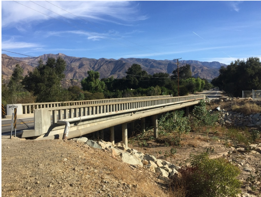
Photograph 1. View of existing pipeline alignment within BSA, facing northeast (Unit A). Photograph shows suspended pipe above San Antonio Creek adjacent to Grand Avenue Bridge. November 13, 2018.
