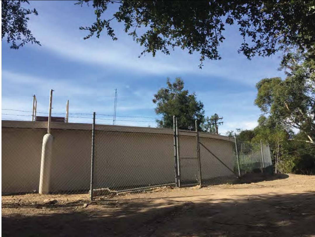
Photo 7. W Arbolada Tank, facing southwest
