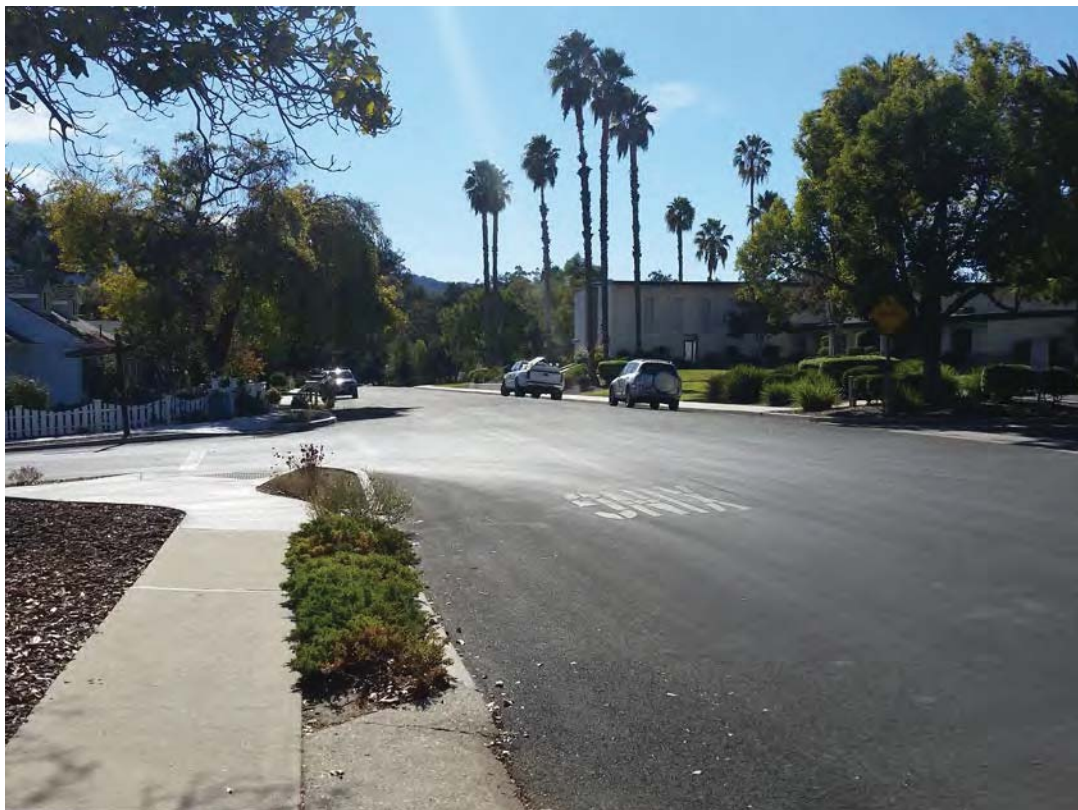
Photo 6. Pipeline alignment on San Antonio Road, facing south
