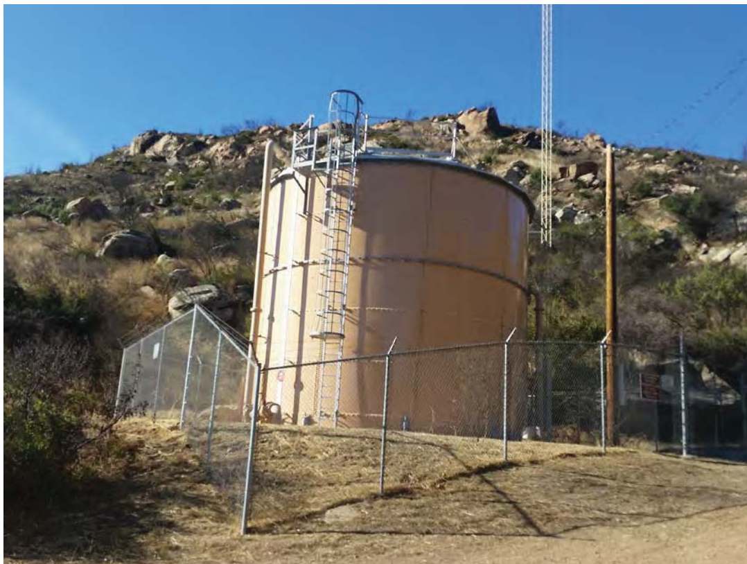
Photo 8. Heidelberger Tank, facing northwest
