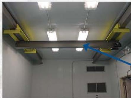
Optional bridge crane for equipment removal.
