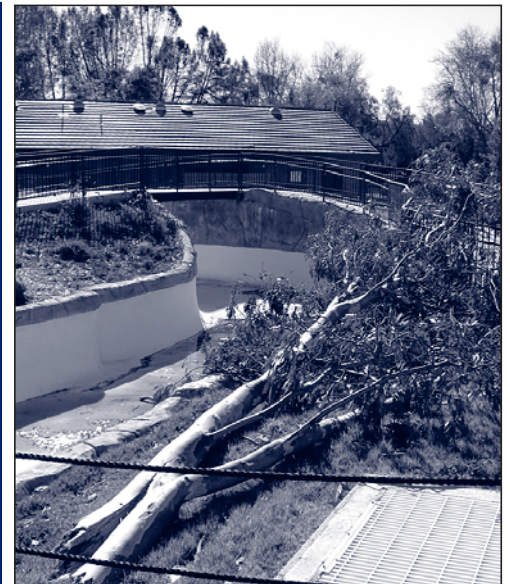
Numerous branches fell near water park.
