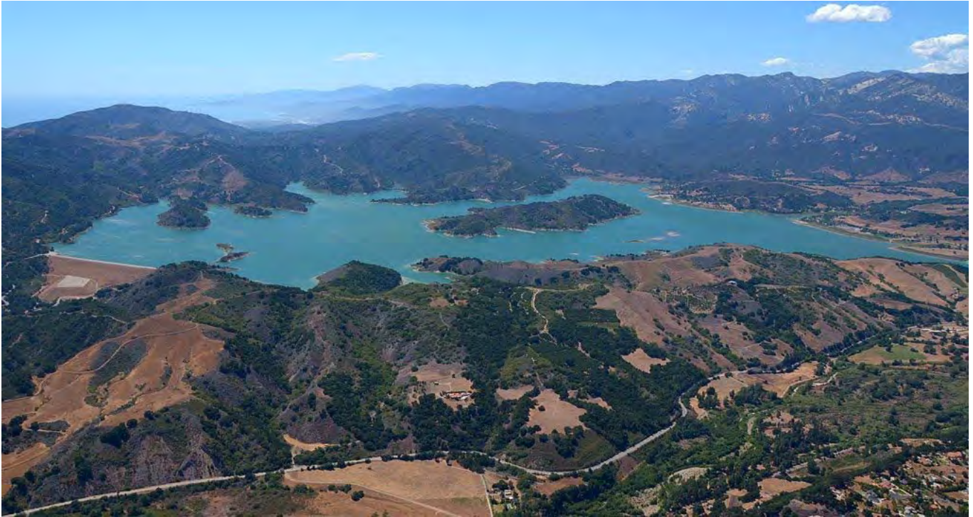
FIGURE 4-2 LAKE CASITAS AND CASITAS DAM
