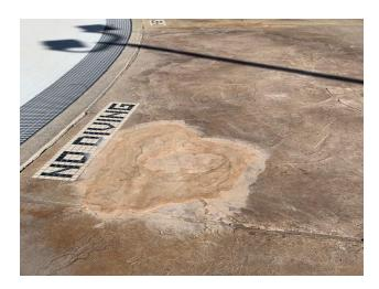
The Casitas Water Adventure staff continued to work on the decking surrounding the Lazy River and Play Structure patching and repairing concrete surfaces, which requires constant attention (picture above). The upgrade and completion of the new Chemtrol chemical controller system will maintain water quality, freeing technicians time to preform other maintenance duties during operation. CWA staff also assist with the maintenance daily COVID restroom cleaning.
