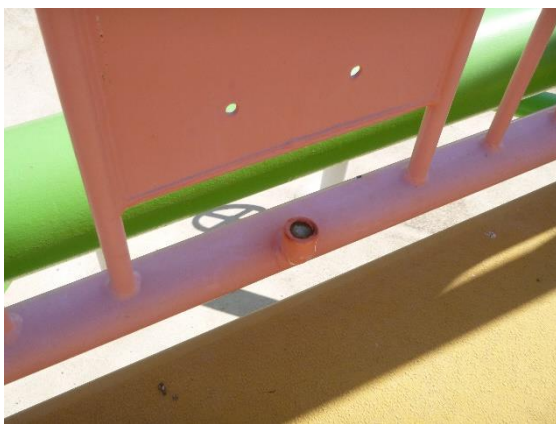
Fig 1.11. Former water gun connection point
