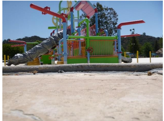
Fig 1.38. Sunken deck around pool
