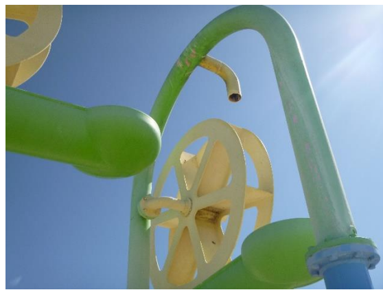
Fig 1.8. Water feature corrosion
