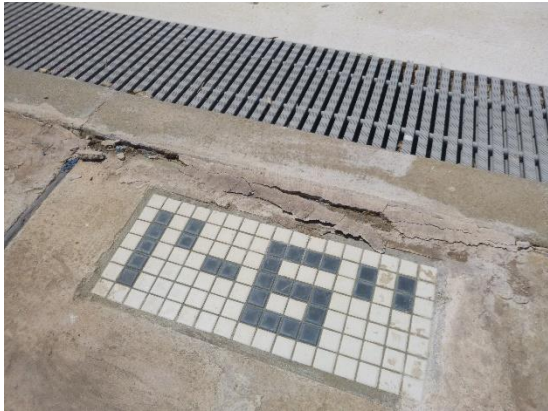
Fig. 1.37. Pool depth marker and joint movement
