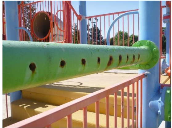
Fig 1.8. Water feature corrosion
