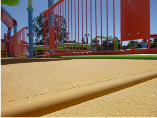
Fig. 1.19. Uneven platform connection
