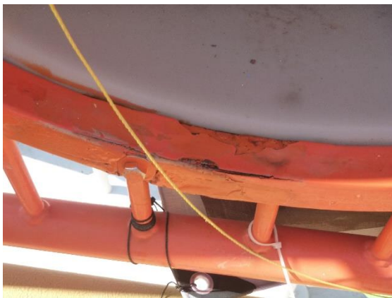
Fig. 1.7. Water feature corrosion
