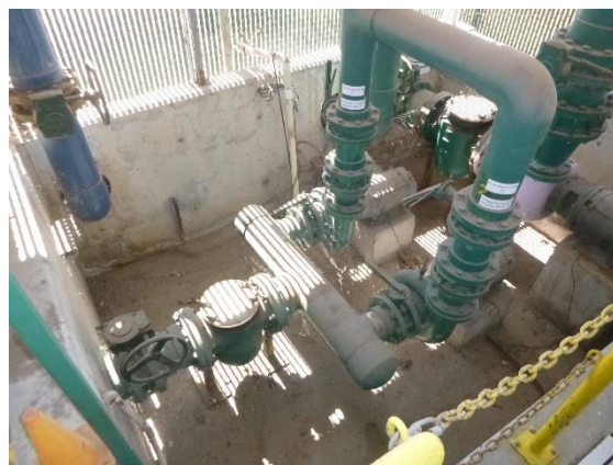
Fig 1.30. Play structure pumps/motors
