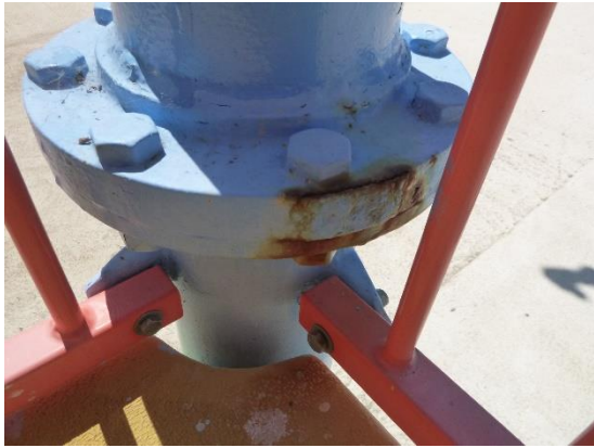
Fig. 1.13. Corrosion on structure
