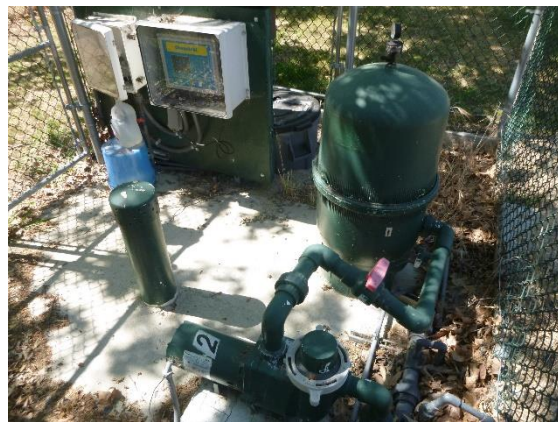
Fig 1.36. Spraypad mechanical system
