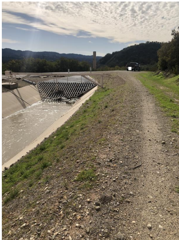
Upper Canal Siphon above OVLC Site
