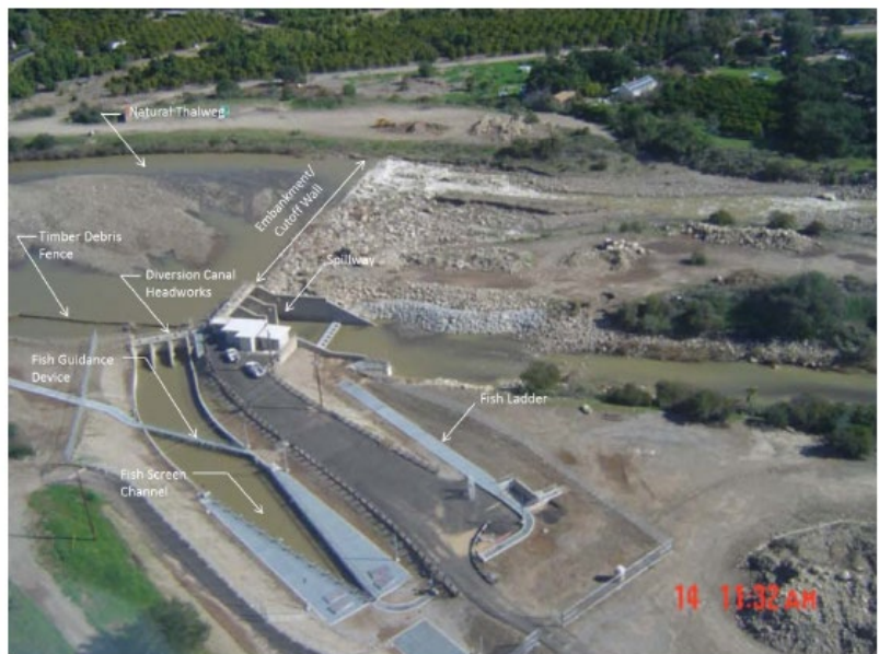
Figure 5-5. Robles Diversion Fish Screen (MKN Associates, 2019)
