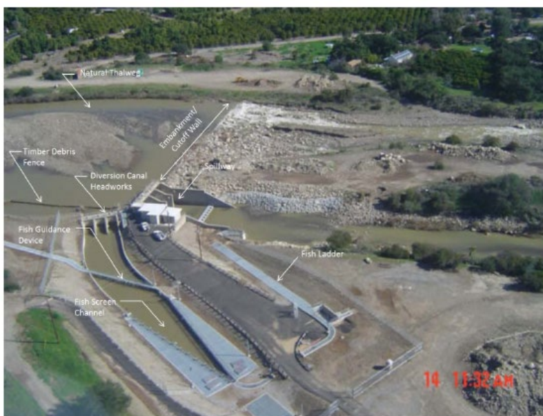
Figure 4-5. Robles Diversion Fish Screen (MKN Associates, 2019)
